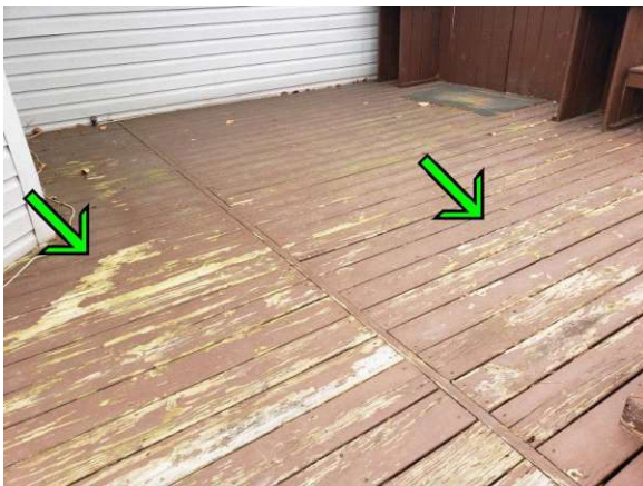
Paint / stain deck surface
