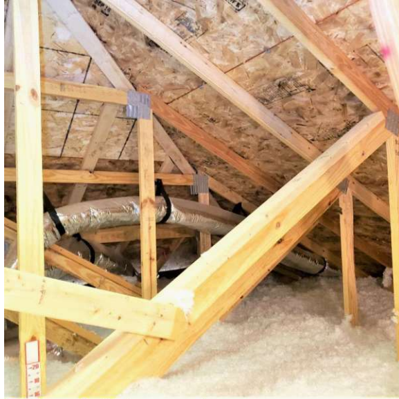
Portion of attic truss system
