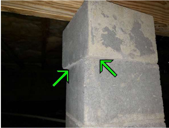
Dry-stacked block on support pier
