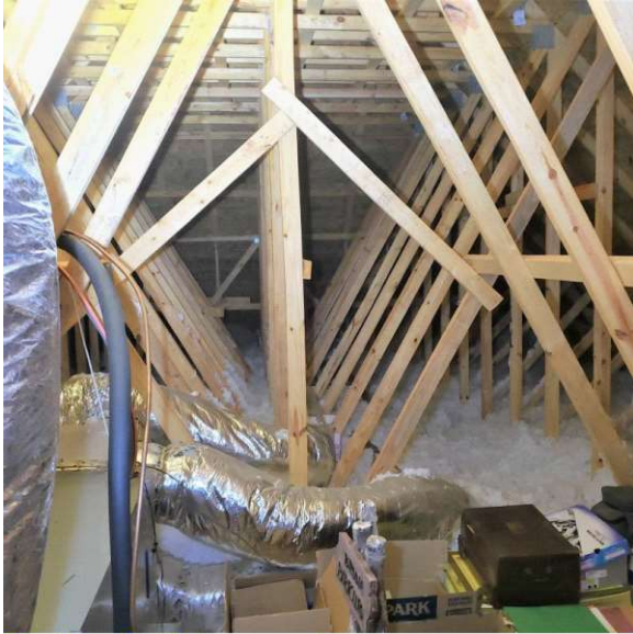
Portion of attic truss system
