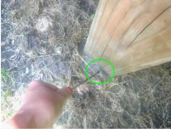
Probing bottoms of support posts
