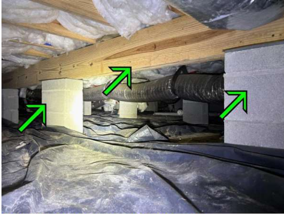
Portion of main beam and supports
