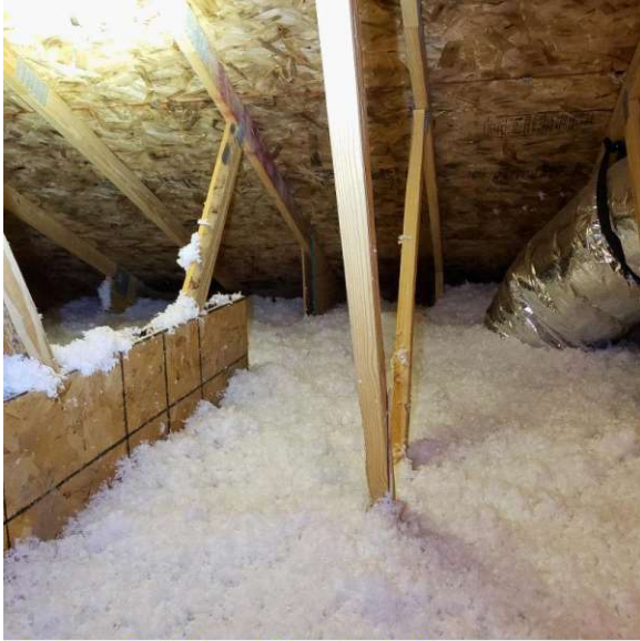
Portion of attic insulation (typical)
