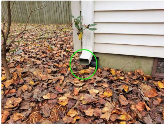
Extend downspout / Right rear
