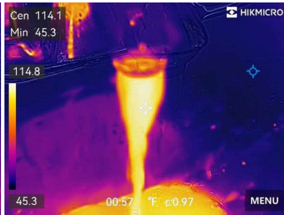
Hall bathroom - 114 degrees F
